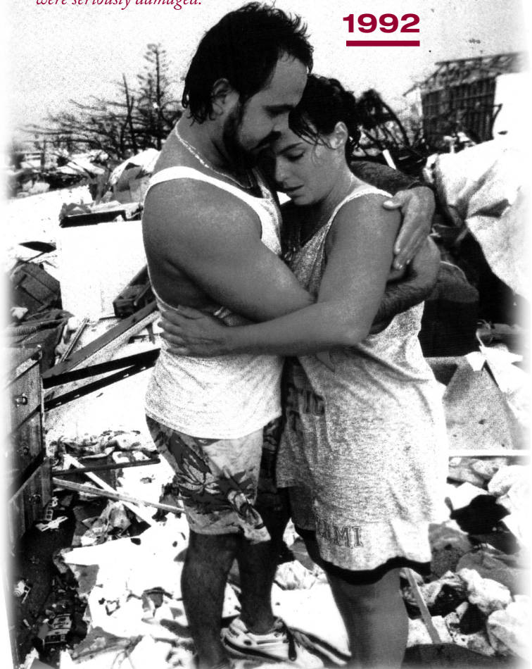
In Miami-Dade County more than 25,000 houses were destroyed by Hurricane Andrew and about 100,000 more were seriously damaged.
